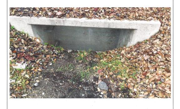
Stormwater drain, directly adjacent to the main building – no screen or barrier Drains directly to Eaton Canyon Wash
