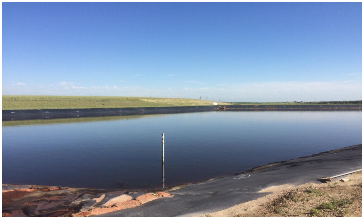
Lined leachate pond with depth gauge.
