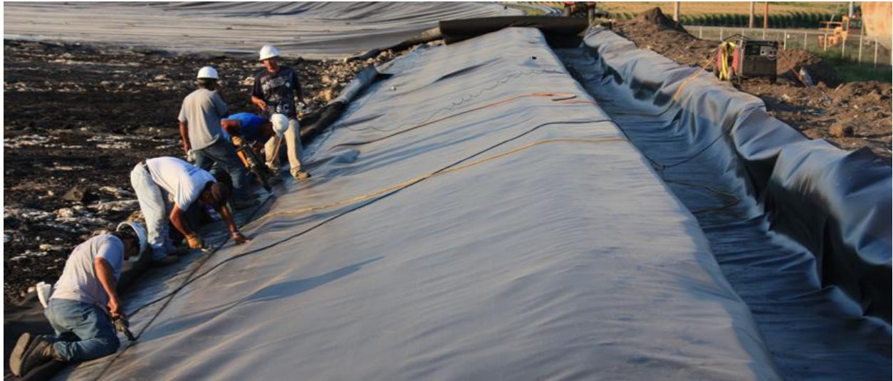
Installation of High Density Polyethylene (HDPE) geomembrane (liner). On the right is an anchor trench, used to fix the liner in place and prevent migration of the geomembrane down the side slope of the cell.
