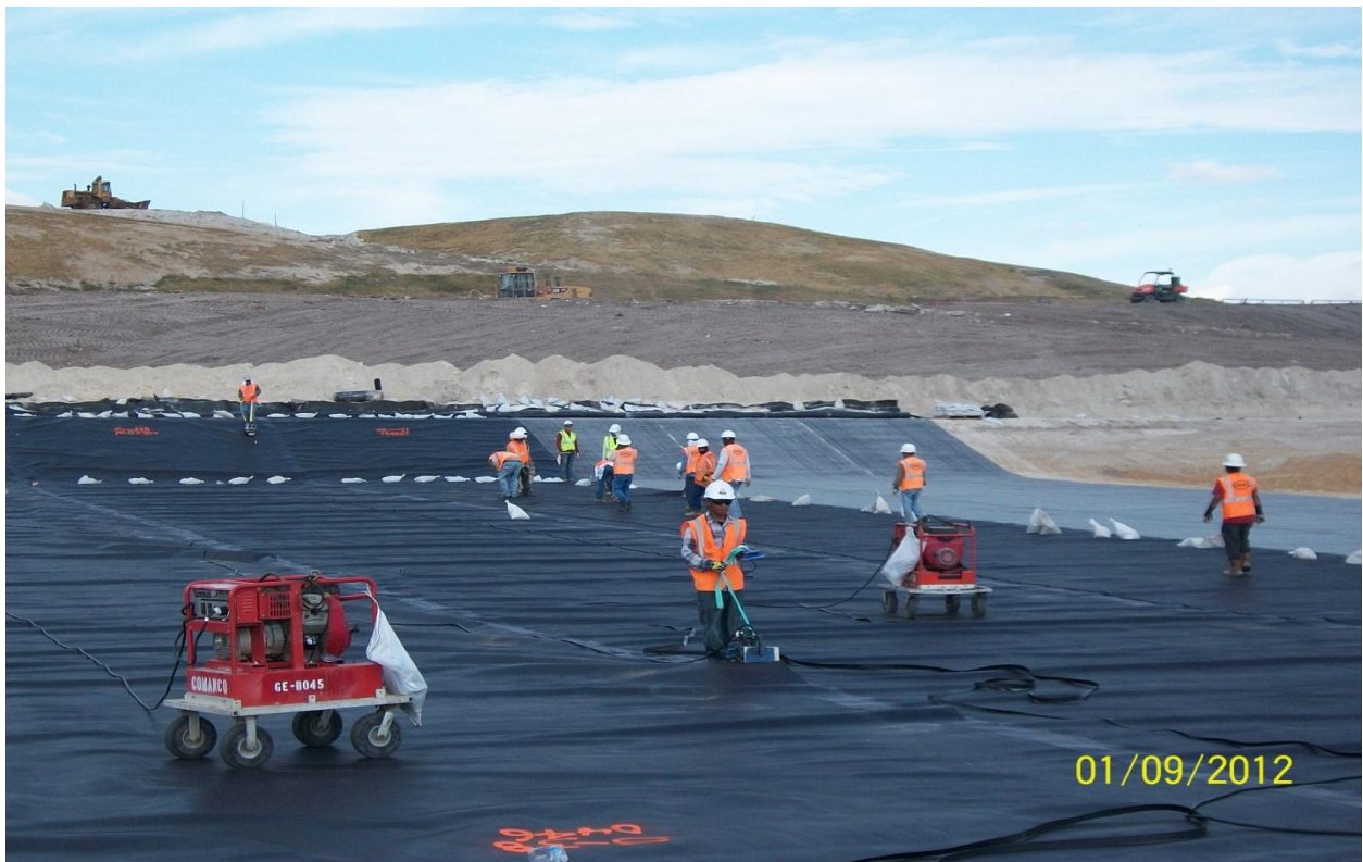
Seam Welding during HDPE liner installation.
