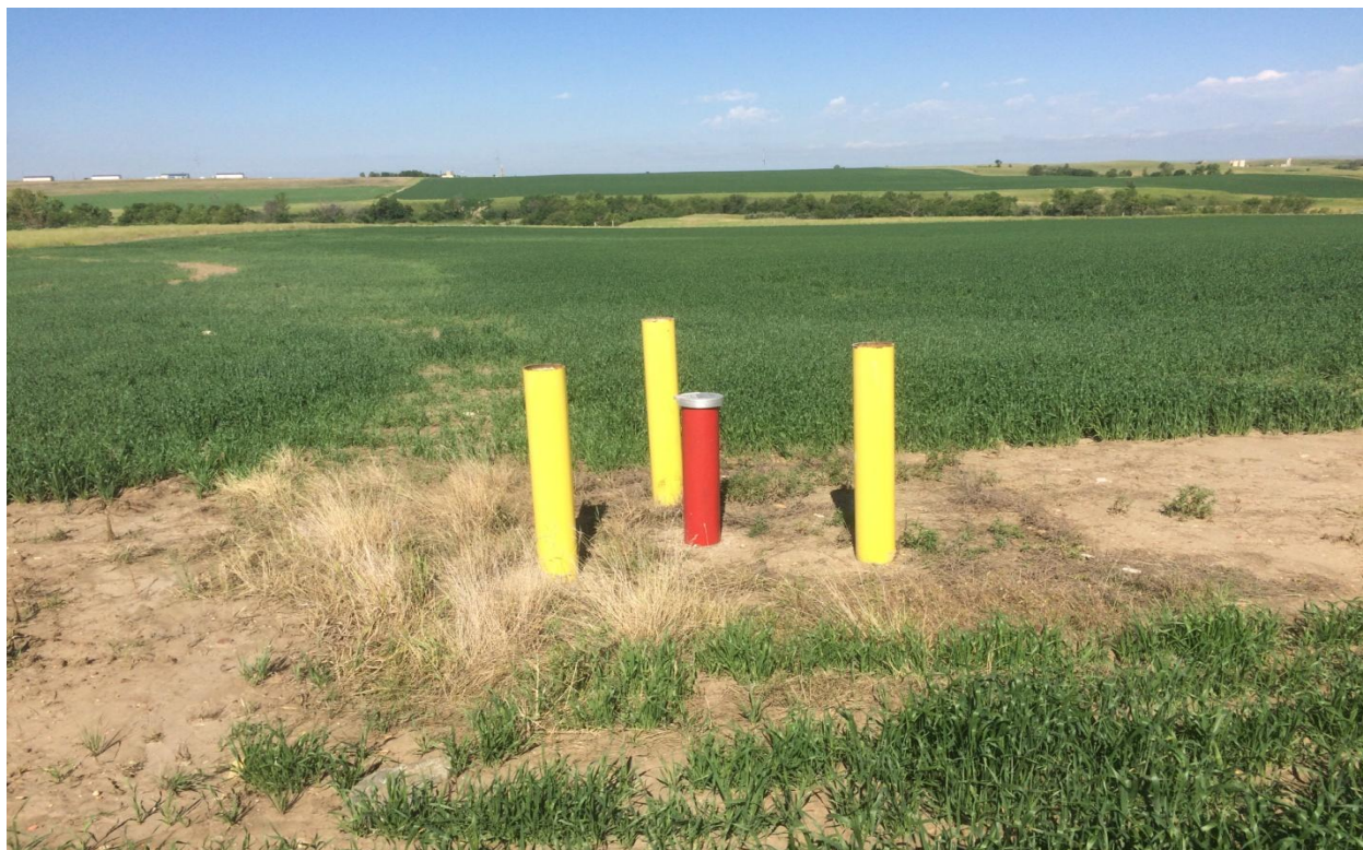
Newer monitoring well, properly labeled and protected with bollards. West of MWU-1.
