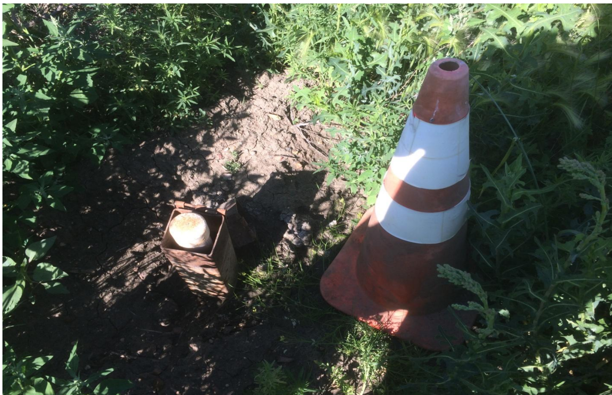
Monitoring Well. Unsecured (no cover or lock), unprotected (no bollards), and hidden by vegetation.
