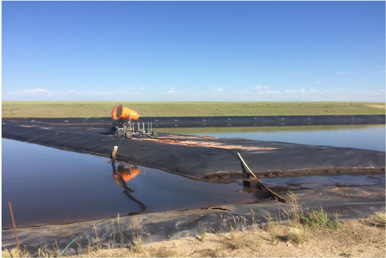
Separation between lined leachate ponds with fan to augment evaporation as necessary.
