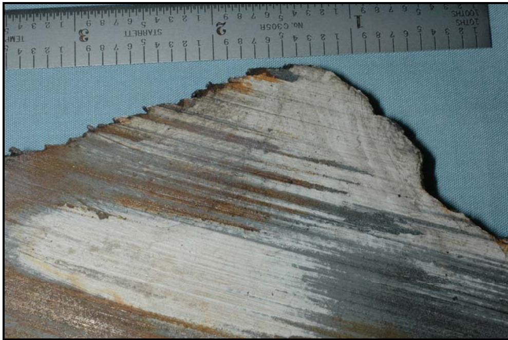
Figure 22: Shows that the cracks on the inside surface have not extended to the outside surface of the tank head.
